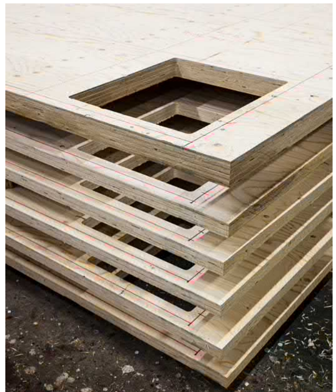
Figure 1.48. Holes in LVL panels.
