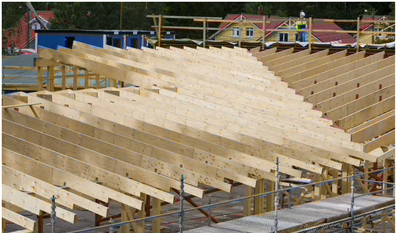
Figure 2.27. LVL-P rafters in a mono-pitch roof structure.
