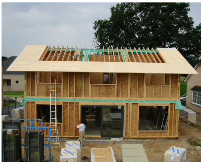
Figure 2.47. Eaves and roof overhangs from LVL-C panels.
