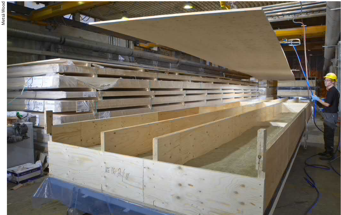
Figure 1.57: Manufacture of structurally glued LVL roof elements.
