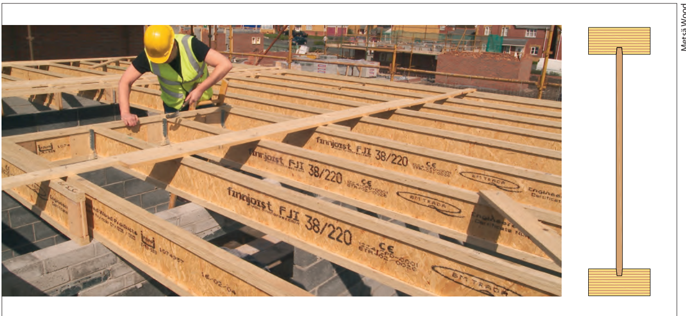
Figure 2.94. Wooden I-joist with LVL flanges.
