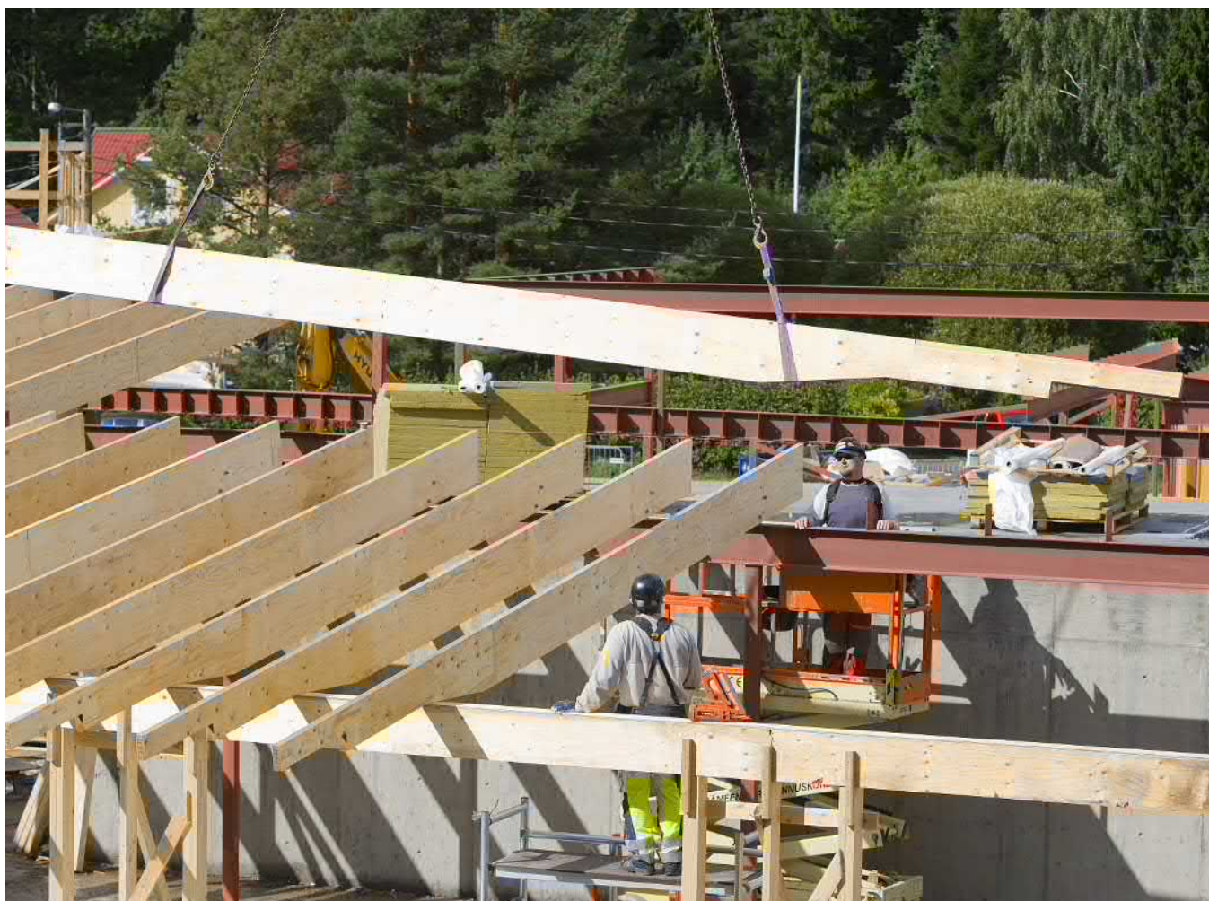
Figure 1.49. LVL-P roof beam cut to special shape.
