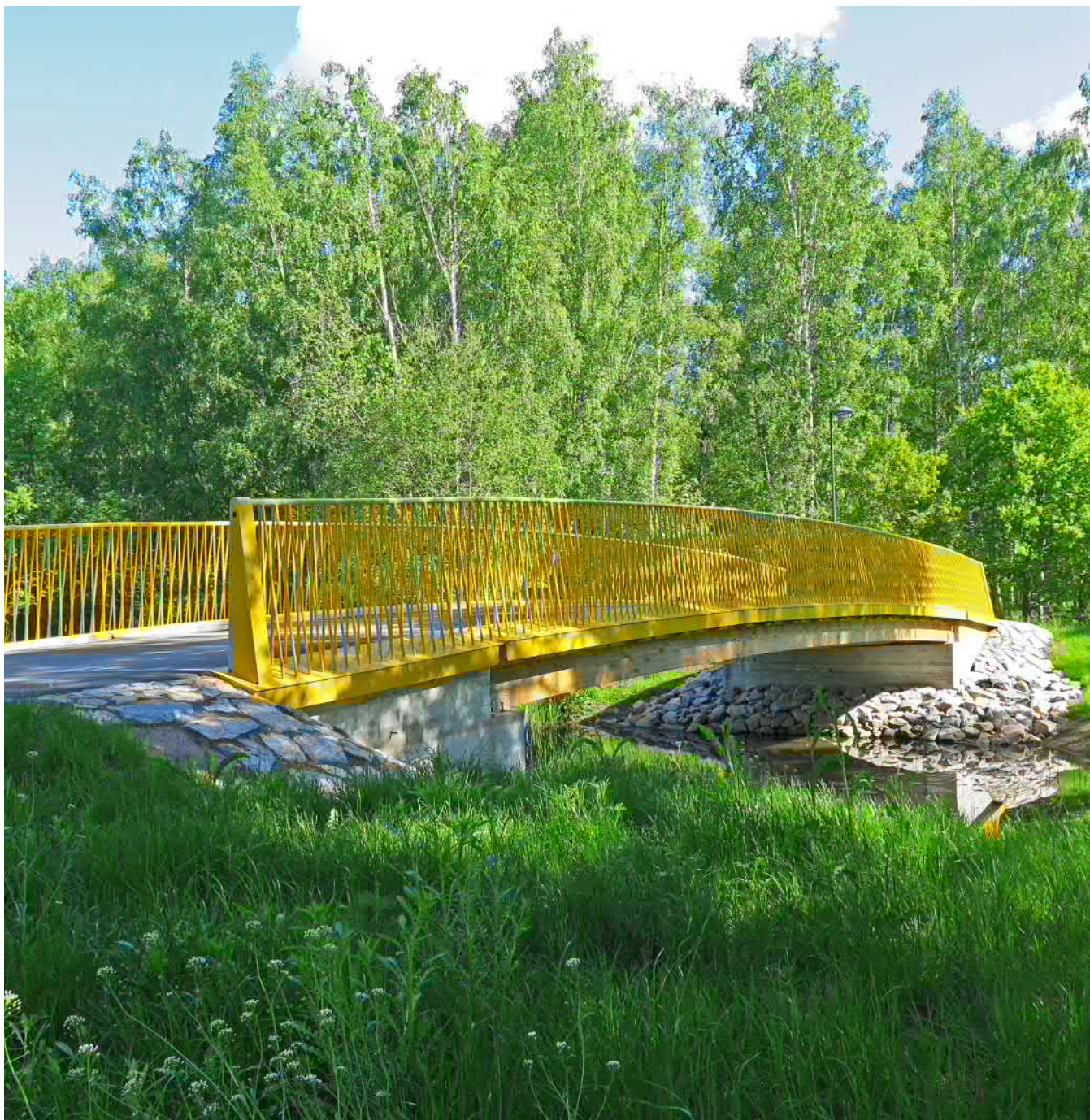
Figure 7.1. Wooden pedestrian bridge, Matinpuron, Espoo, Finland.
