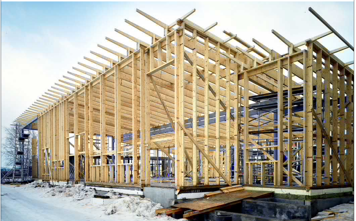
Figure 2.58. LVL-P studs for tall load-bearing exterior walls.
