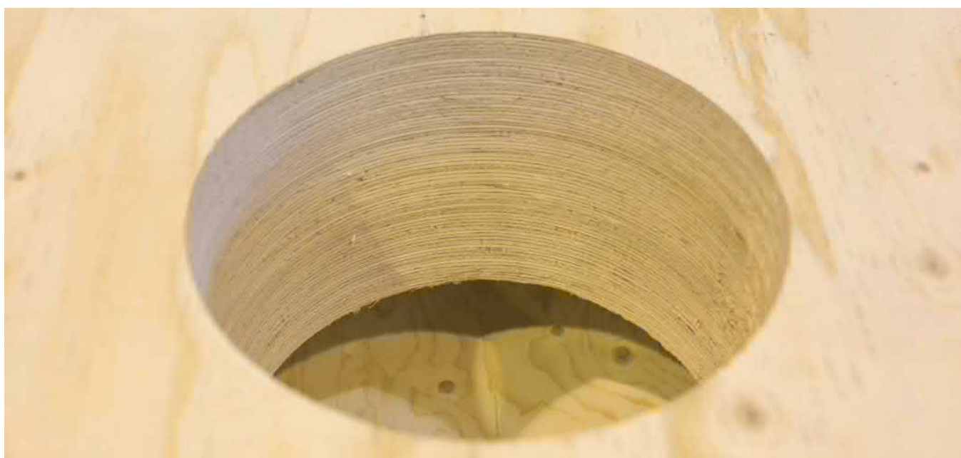
Figure 1.50. Hole in an LVL beam.
