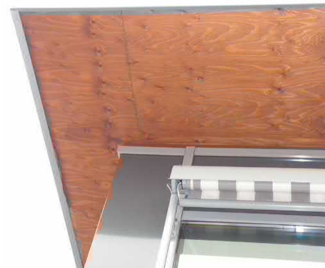
Figure 2.48. Surface treated eave panel.
