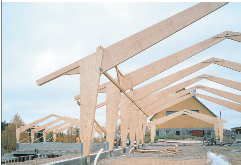
Figure 2.83. 3-pin portal frame structures for hall constructions with moment-resistant bolt circle corner connection.
