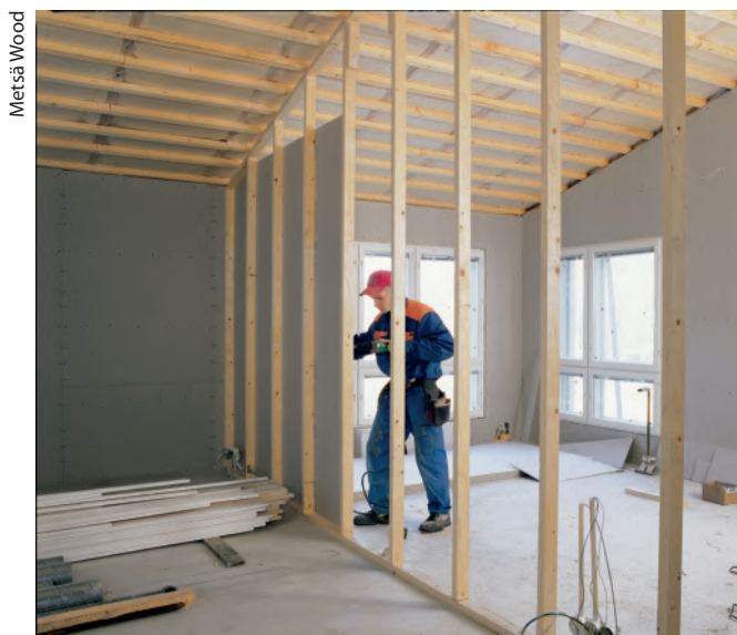
Figure 2.56. Installation of plasterboards to LVL-P wall studs.
